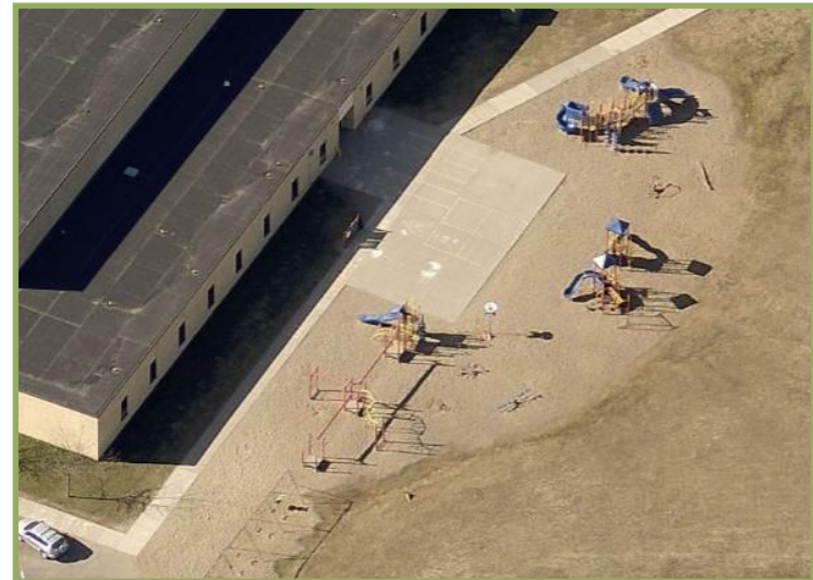
Figure 25: Stanley Elementary Playground.
